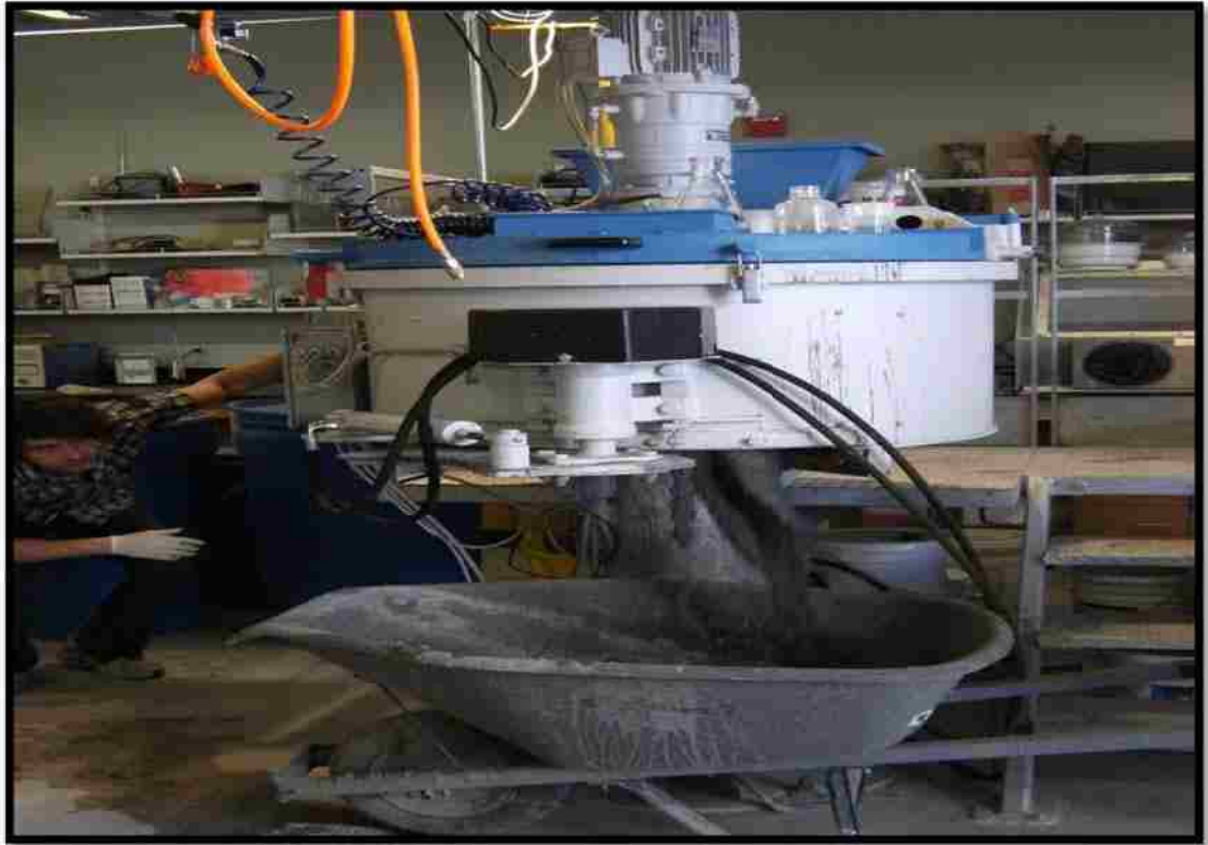
Figure 3.2: The final mix exiting the mixer
